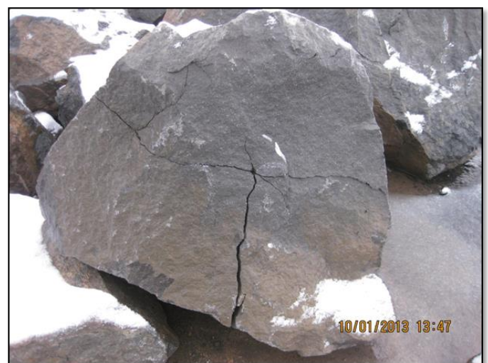
Figure 11. Fractured riprap stone in site test
