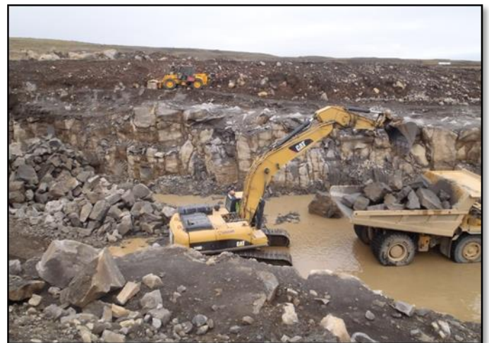
Figure 3. Excavation of basaltic lava in the Approach Canal
